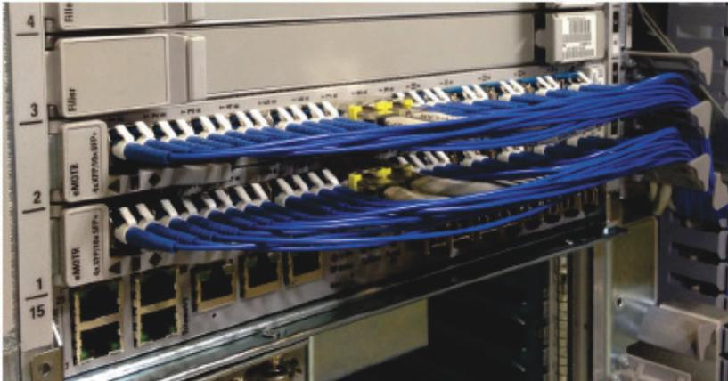
Route CAT5 cables behind fiber; two cables per fiber manager.
