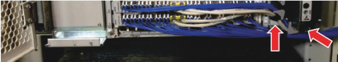
CAT5 cables can be secured to the bottom of the lower fiber manager and routed towards the back through the shelf side air intake.
